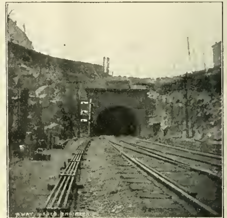
EASTERN PORTAL OF BERGEN HEIGHTS TUNNEL, NEAR NEW YORK, ON THE ERIE RAILROAD.
